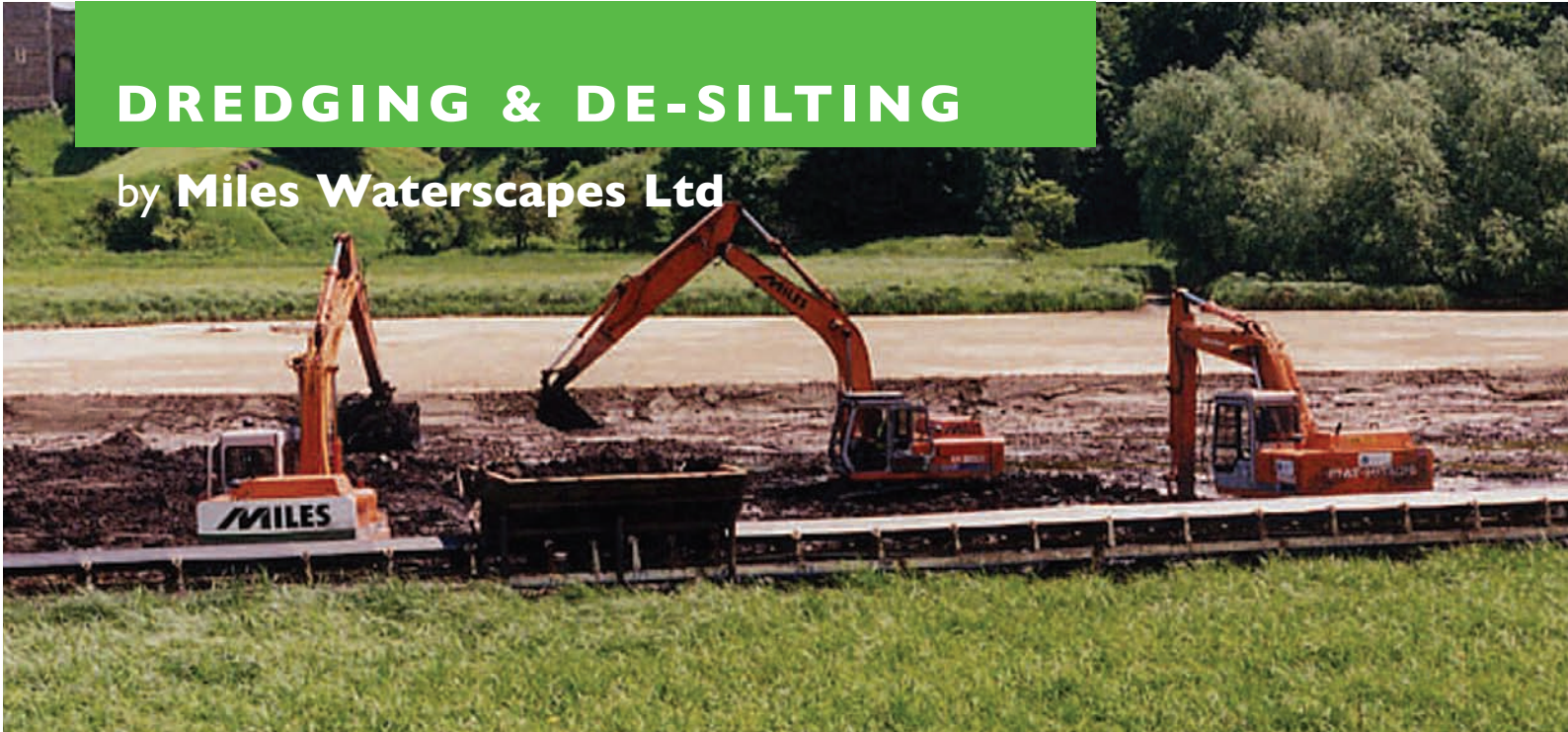
Removing unstable soils, vegetation and silts from Framlingham Mere.
